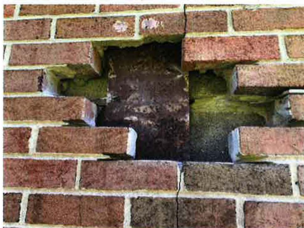
Figure 4 – Exploratory Opening at the West of the Nave (Location 4)
