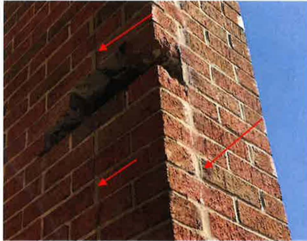
Photograph 2 – Observed Cracking along a Column
